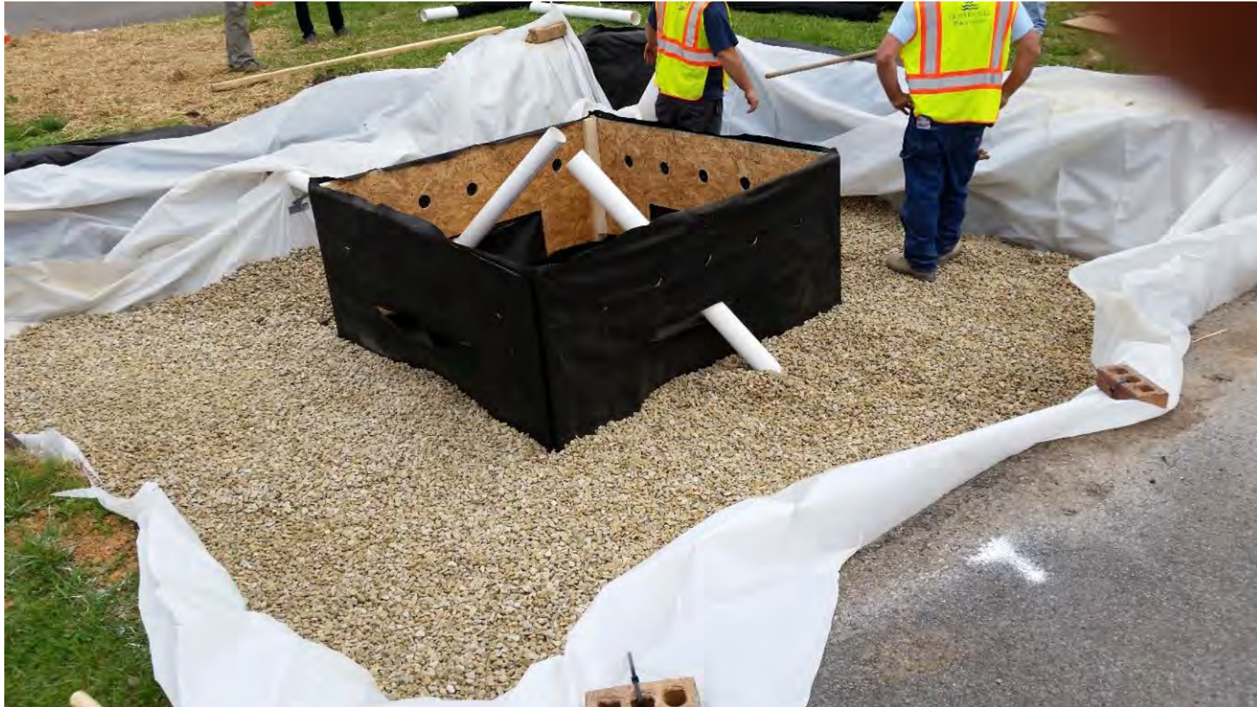
Quartzitic Sandstone – 0.75" Crushed Stone 4 ply, 6 mil clear plastic sheeting to hold water in system
