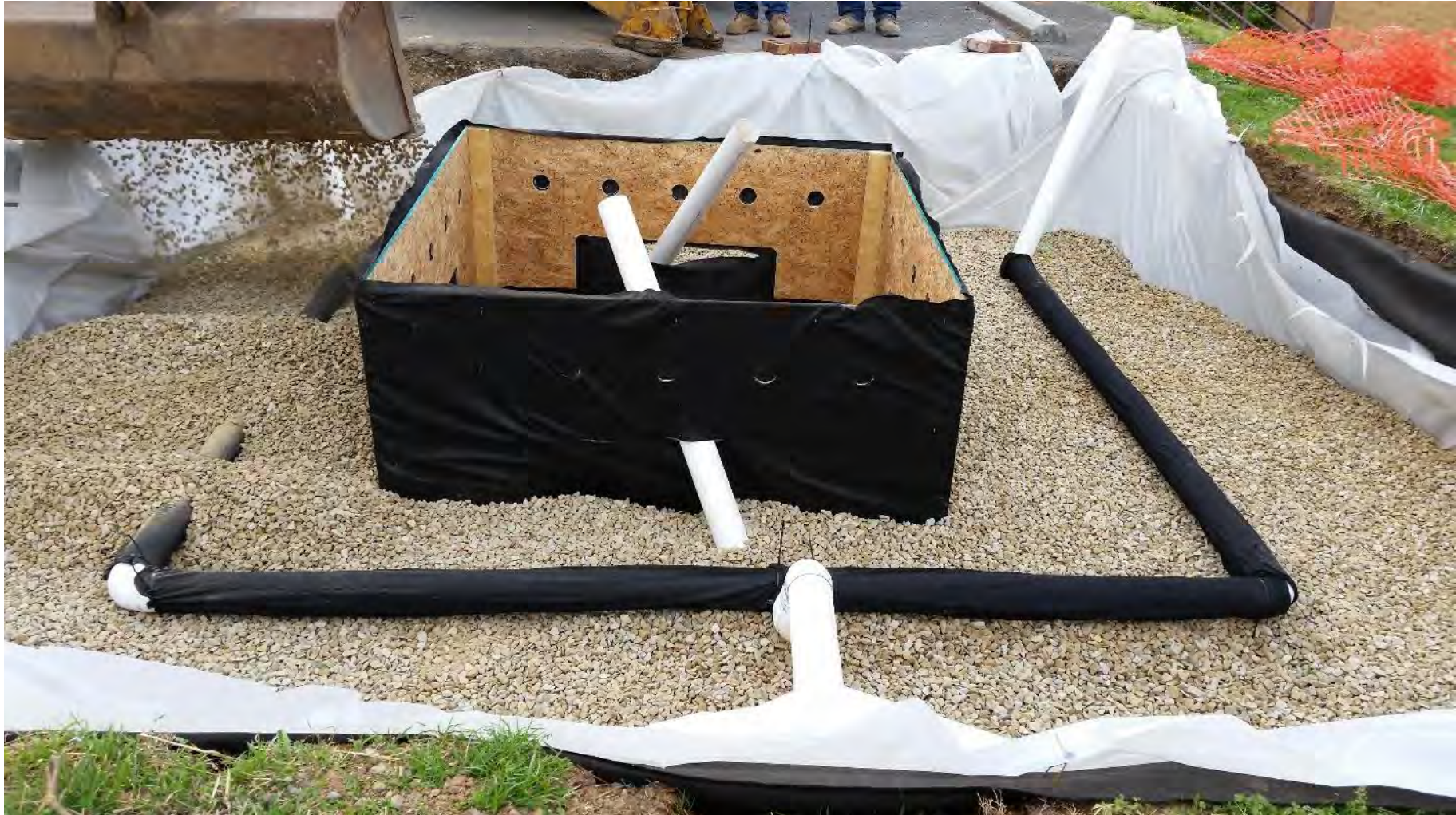
4" perforated PVC sewer drain pipe with up-turned elbow Under-drain in place with black drain sleeve
